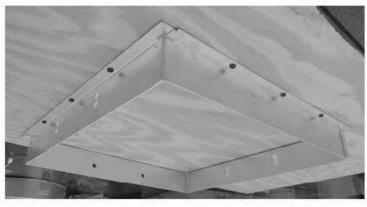
Attach mounting ring to wood sheet or strips with  $\frac{1}{2}$ " wood screws Make sure frame is mounted square
